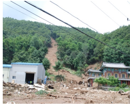
(b) Steep slope failure
